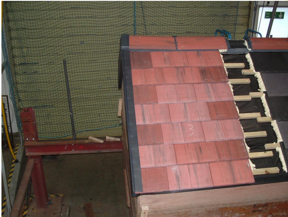
Figure 1 Manthorpe SmartVerge® Linear Dry Verge System - left verge with plain tiles (verge 3)
