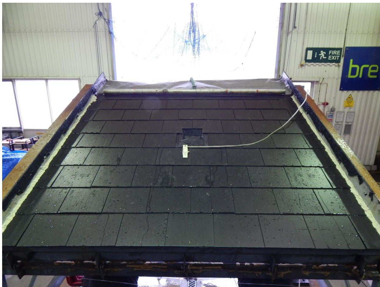
Figure 2 Small Format Slate Vent installed with Fibre Cement Tiles
