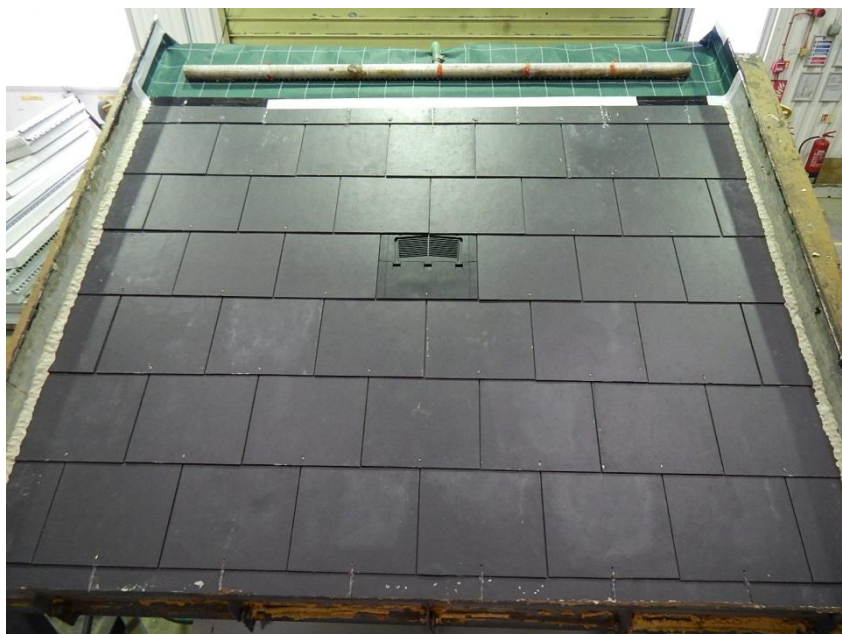
Figure 1 Vent slate installed on the roof
